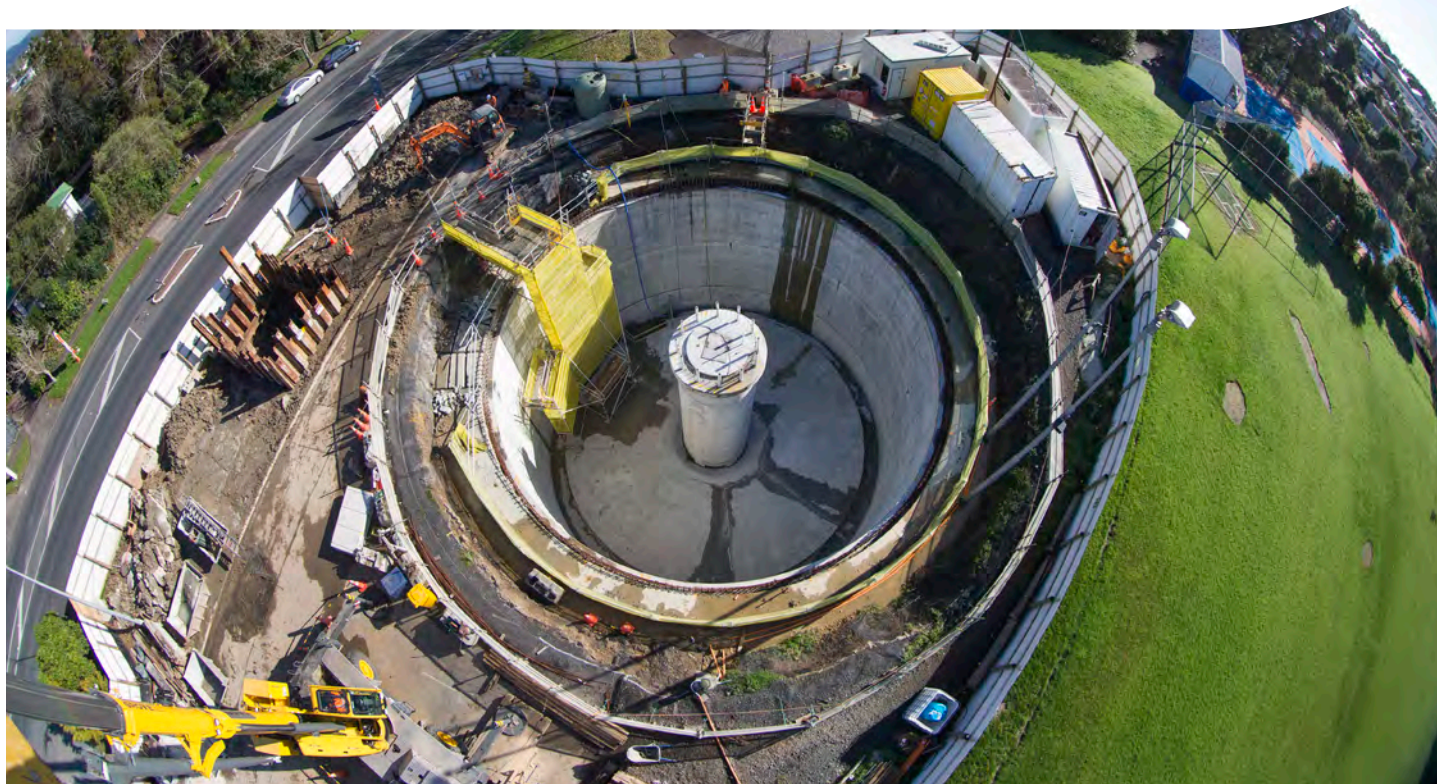
The concrete storage tank at Harold Moody Reserve.
