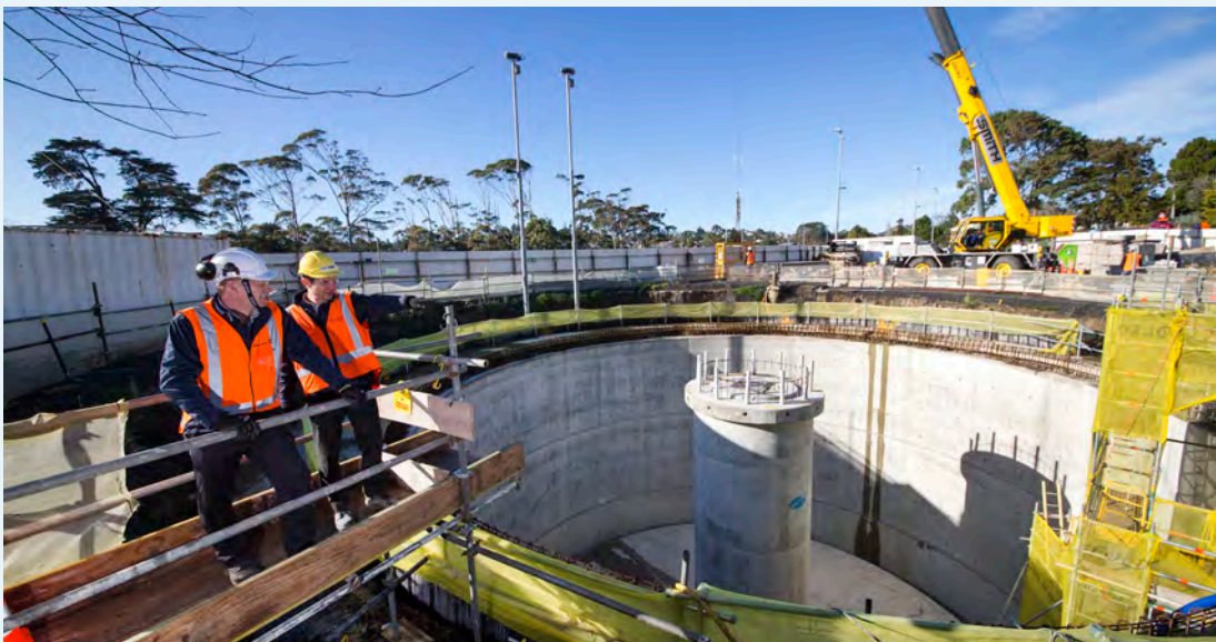
Watercare's project managers James Eardley (left) and Peter Kukulsky inspect progress.
